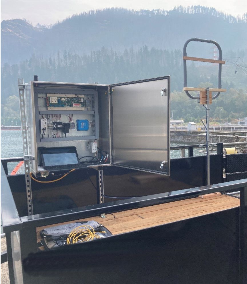
Bonneville Dam PH1 Radio Frequency Interference Monitoring Station
