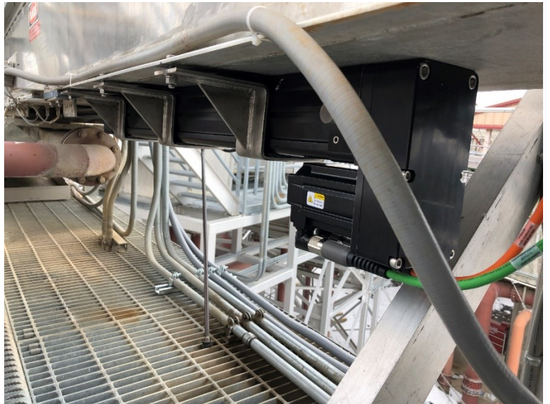
New Electric Cylinder at LMJ A-B-Side gate.
